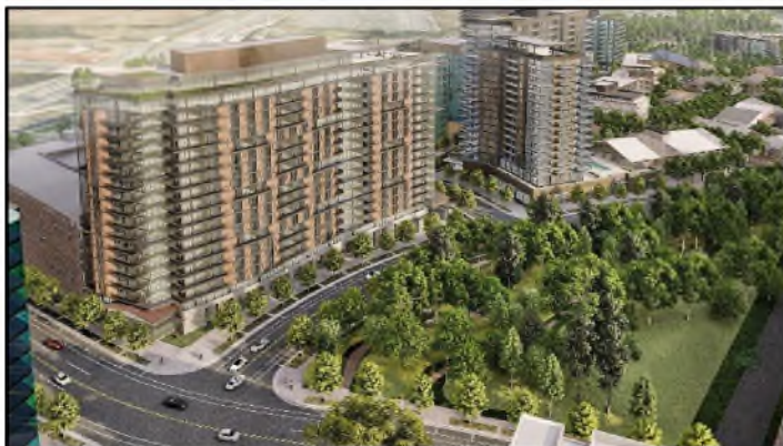
Rivana at Innovation Station - Highrise Multifamily
