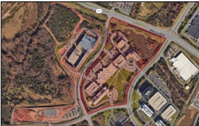
Pacific Corporate Park - Existing Conditions
